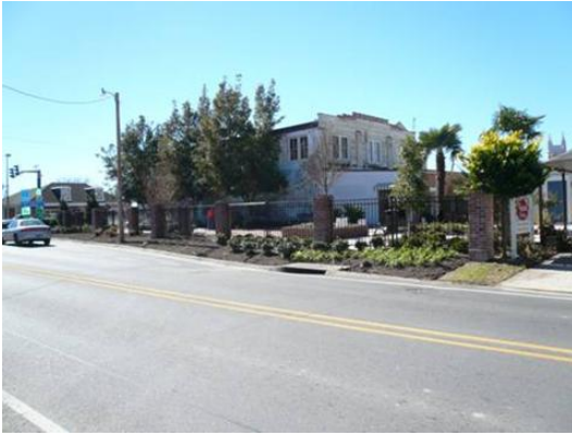
Figure 8. This facility has been completed and is in use.
