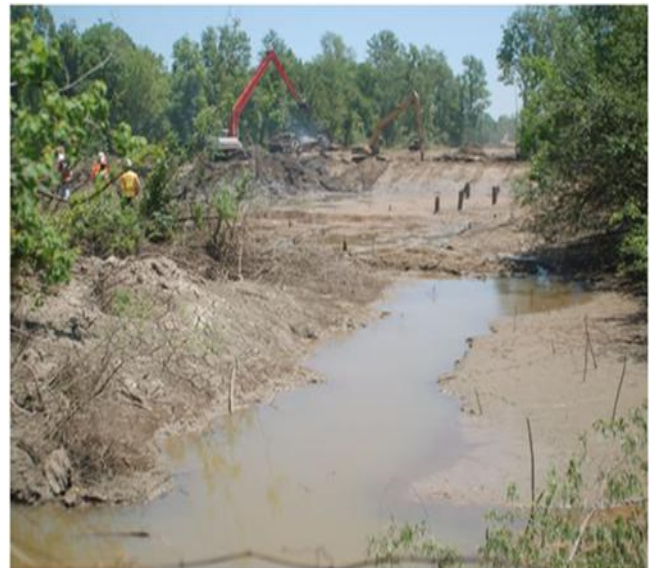
Figure 2. Element 9-2 constructed at Buffalo Cove
