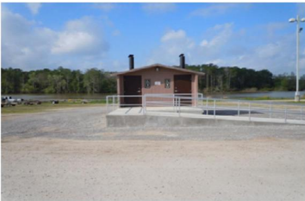
Figure 6. Modular restrooms now operational.
