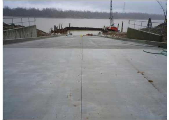
Figure 3. Construction has begun on the Krotz Springs Boat Launch
