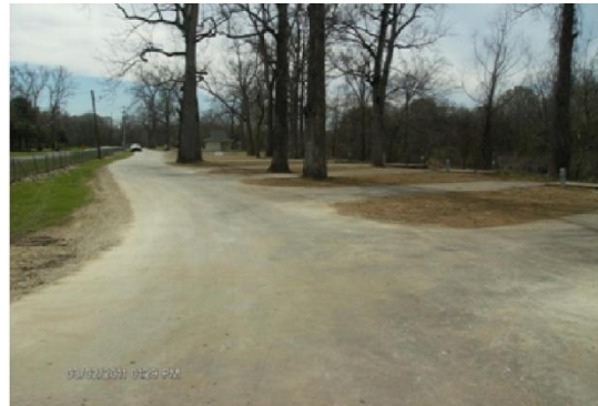
Figure 9. Construction completed on Dick Davis Park, Phase II.
